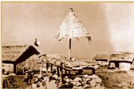
A Post located in the river bed of Brahmaputra
