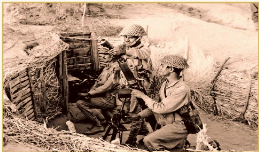
BSF Mortar Det in Action
